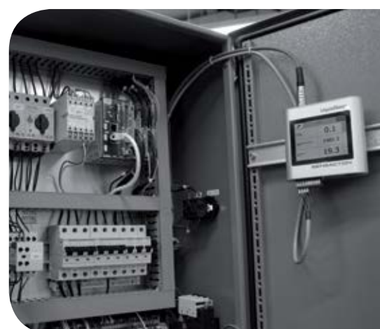
Above image: LiquidSens Controller Touch in the control cabinet of a cleaning system
